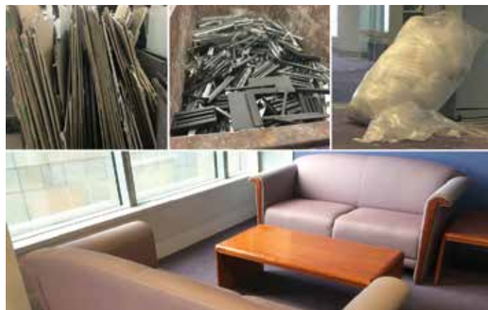
Clockwise from top left, the materials for removal separated – plasterboard; metals; insulation; example of the furniture recovered from GMT.
